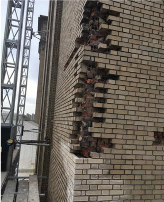
Tower brick replacement, north elevation west corner.
