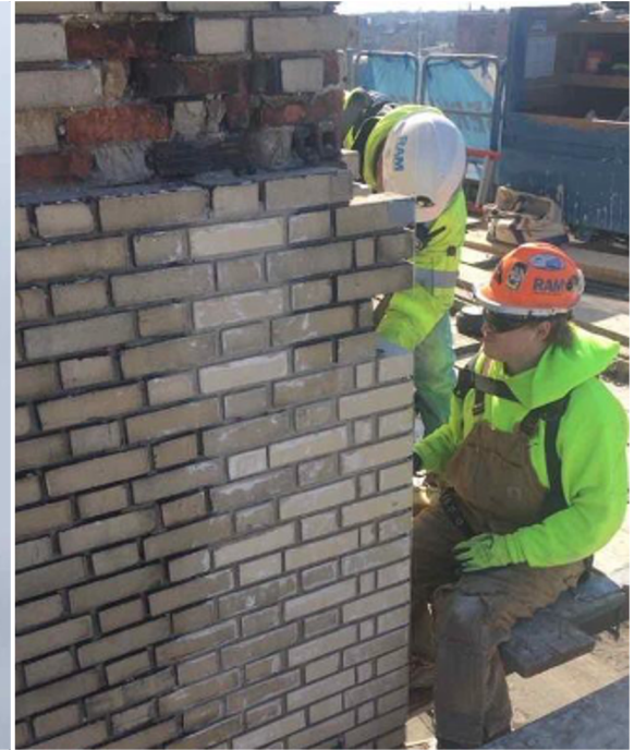
Tower brick replacement, southwest corner.
