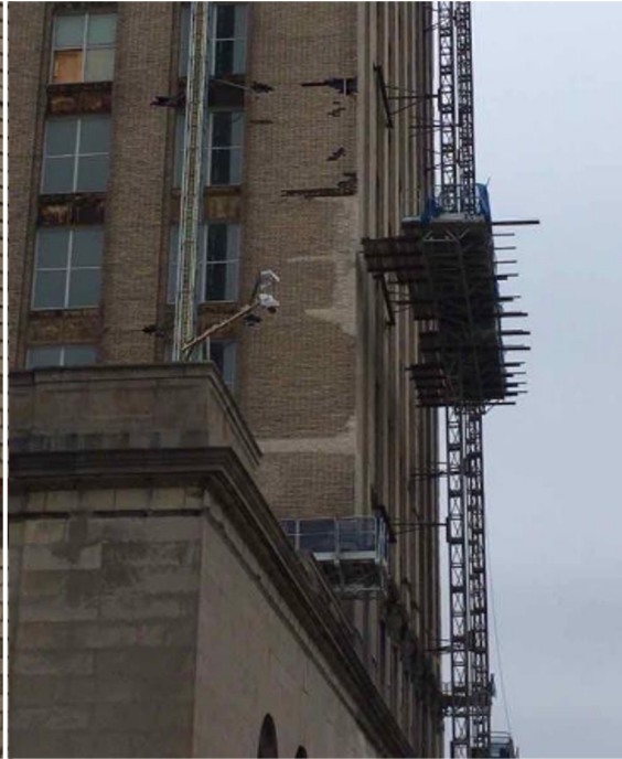
Tower brick replacement, northwest corner.
